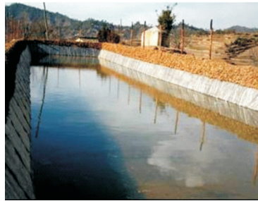
Fig. 6. LDPE film lined tanks at Darim
