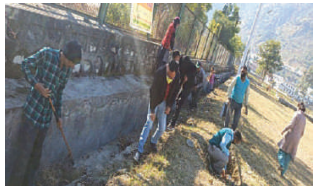
Cleaning of sewerage and water lines & waste management activities
