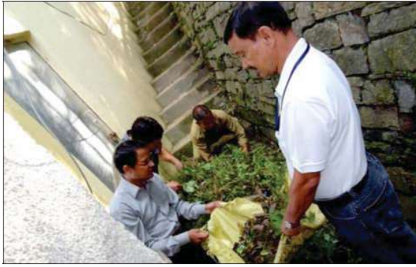
Cleaning the backside of institute office building
