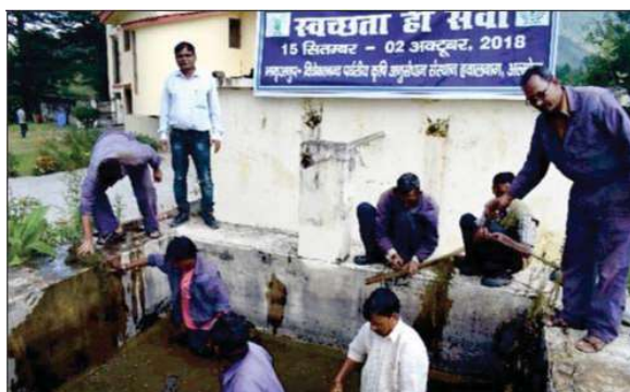
Cleaning of water tanks at Hawalbagh campus
